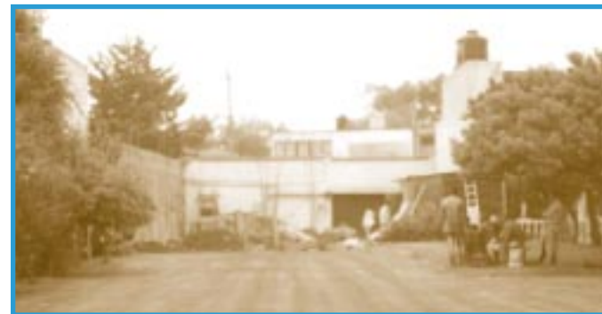
Beginning of Construction Project in Mexico City
