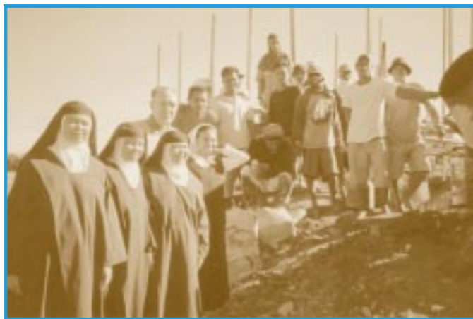
Construction Workers at Monastery in Tarlac
